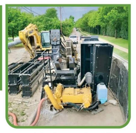
P.E., to engineer a plan that would not only succeed but also give a margin of error that would satisfy everyone. For noise cancelation we encircled all equipment with fencing and ECHO-BARRIER noise reduction matting to maintain the requested decibel level or below at all times. To provide adequate drilling mud management, a Tulsa Rig Iron MCS-355 reclaimer was utilized, as well as in-house 130BBL vacuum trailers for disposal.
